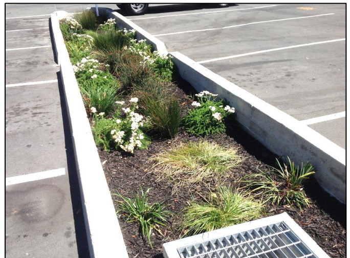
A LID bioretention facility constructed to meet post-construction stormwater control requirements. Photo courtesy of the City of Santa Cruz.
